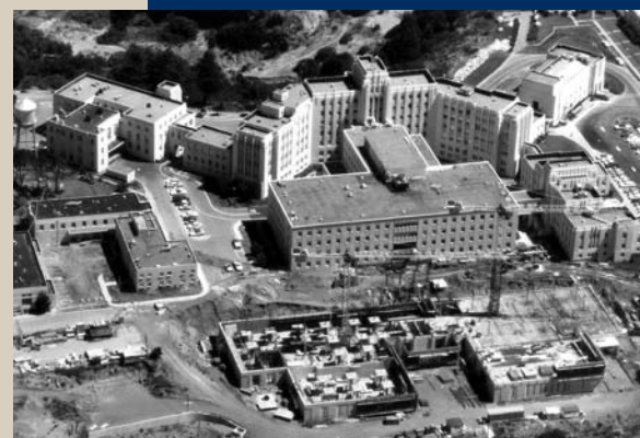
Construction of Building 203 began in 1973.
